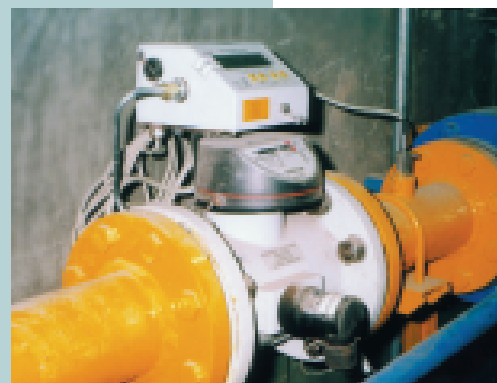
Turbine meters with EK-90/K.
